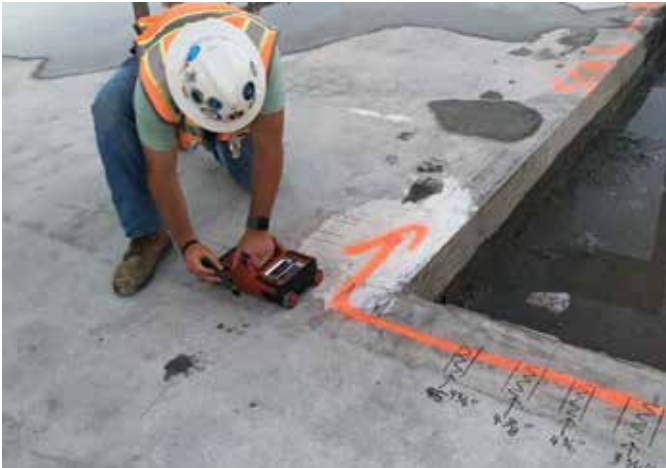
Fig. 4: Location of PT cables were marked
